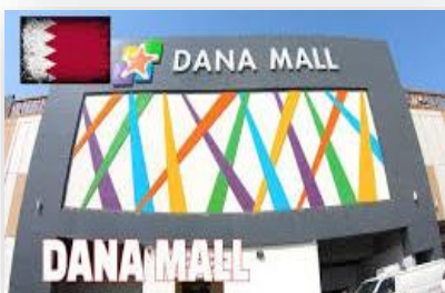
DANA Mall Renovation work
