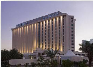
Closing of mezzanine floor @ Sheraton Hotel
